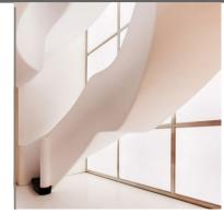
The panels are supplied with an aluminium grid to screw on wall as each of them was positioned inside a cell and blocked with IRON OMEGA ( supplied by Backlight ). All systems were magnetically covered by finish prolfiles ( supplied by general contractor or Backlight).
