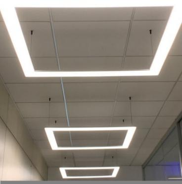
The panels were suspended by Steel Cords which were hanged on the existing. No mounting system can be seen on the lighting surface.
