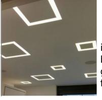
The panels have magnets integrated on the rear side and iron place ( custom bended ) in order to go flush with the false ceiling.
